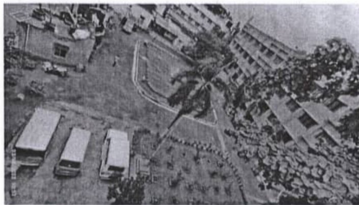
Fig 7.1 Road within campus
