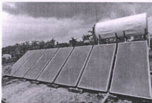
Fig 4.2 Solar Thermal Hot Water System
