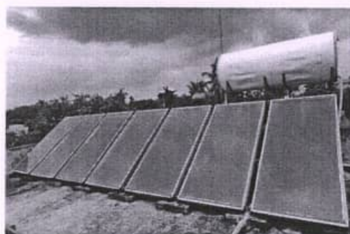
Fig 5.2 Solar Thermal Hot Water System
