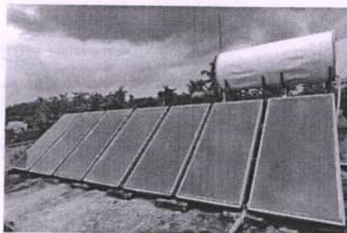
Fig 5.2 Solar Thermal Hot Water System
